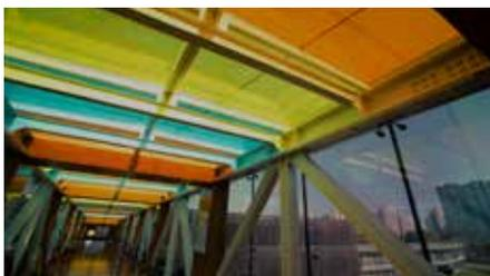
**An example of coloured thin-films for solar energy generation, courtesy FG Glass**
